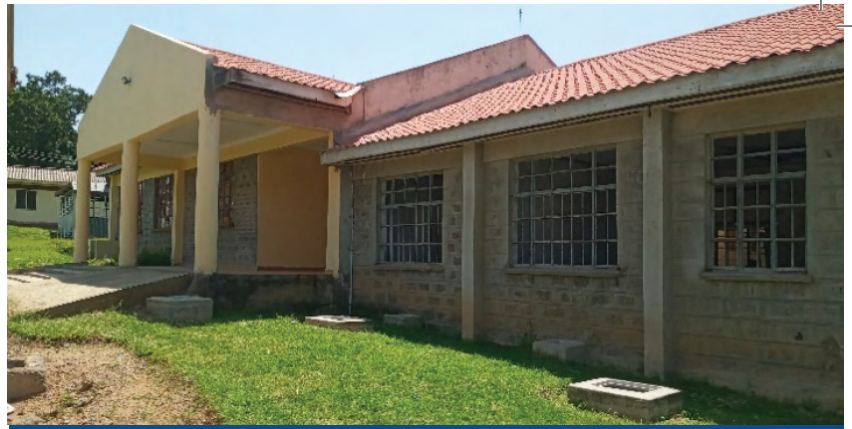
The new general wards under construction
